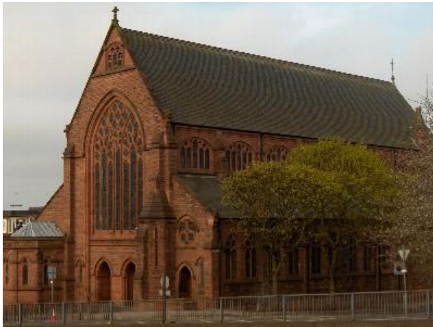
The Church, designed by Peter Paul Pugin is built of Locharbriggs Stone.
